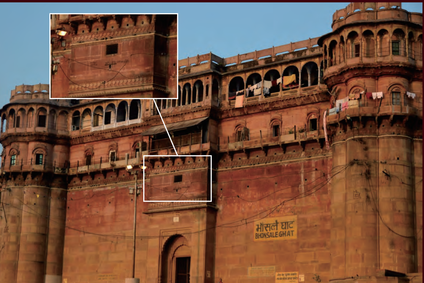
Building along Bhonsale Ghat with Highest Flood level of 1978 marked Inset – Highest flood marking of 1978
