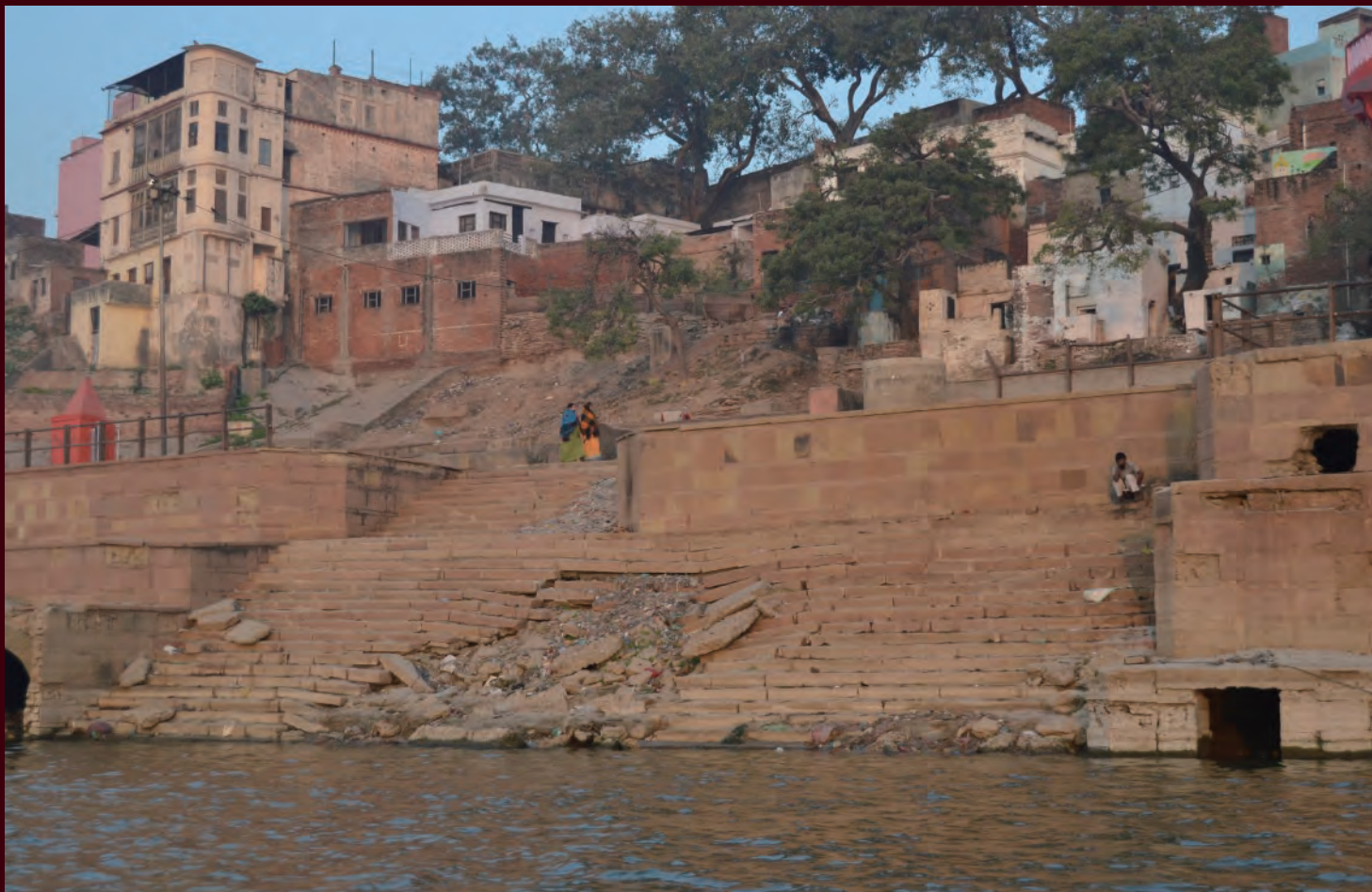
Damage caused to the Ghats by flooding and riverine erosion
