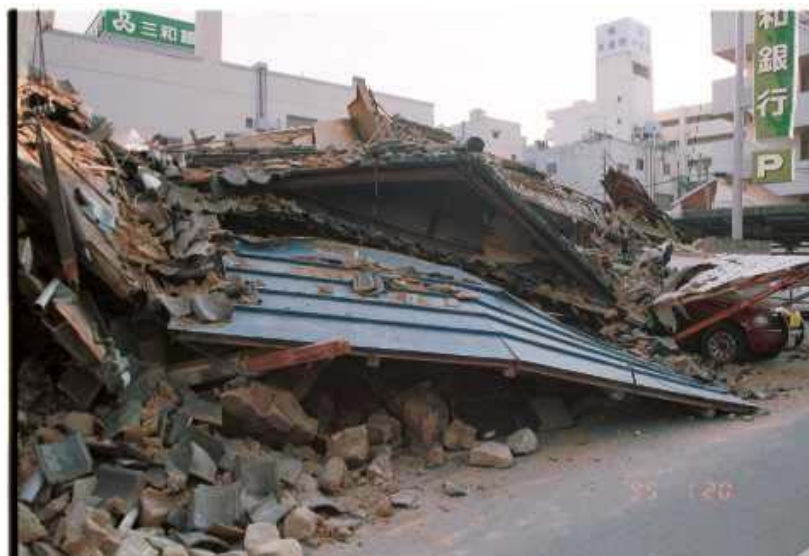
Figure 4.4 Damages of Kobe earthquake (Old wooden buildings)
