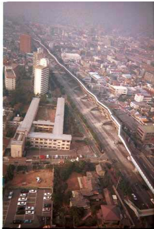
Figure 4.6 Damages of Kobe earthquake (highways)
