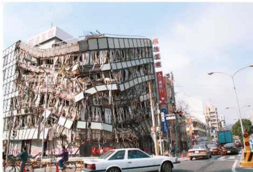
Figure 4.3 Damages of Kobe earthquake (RC buildings)
