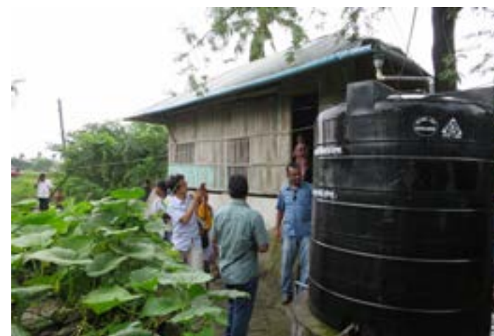
Figure 2. Water tank to collect rainwater
