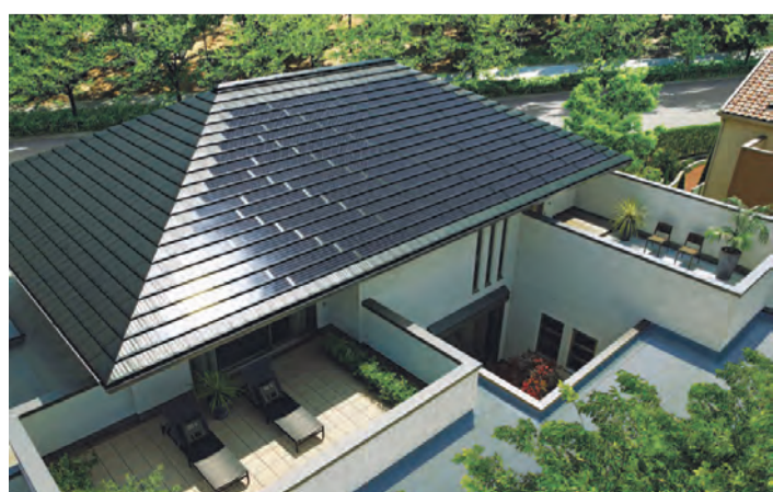
Sekisui House Ltd.'s roofing uses photovoltaic generation technology to address energy needs. SEKISUI HOUSE LTD.
