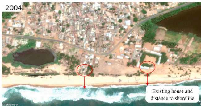
Fig. 8. Location of building to sea (2004). Source: Google Earth
