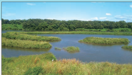
Wetland created for flood control in the Hino River, Fukui, Japan
