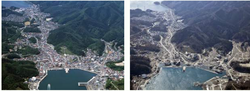
Central area of Onagawa Town, before and after 2011 disaster (Image source: Onagawa Town Hall)
