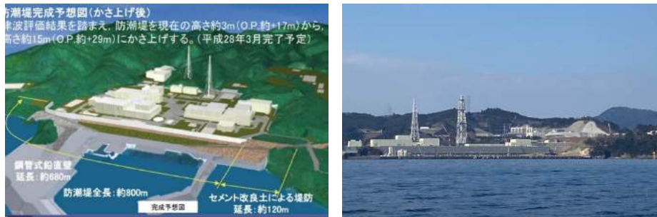
left) Enforcement of sea wall (Image source : Tohoku Power) right) Onagawa Nuclear Station
