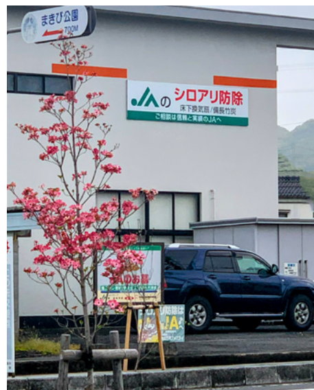
PICTURE 7: Example of orange line (showing the maximum height of water the levees can stop)
